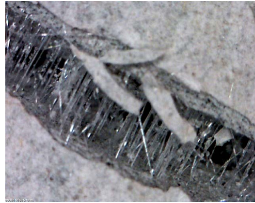
Figure 14: PA66 fibers bridging crack.
